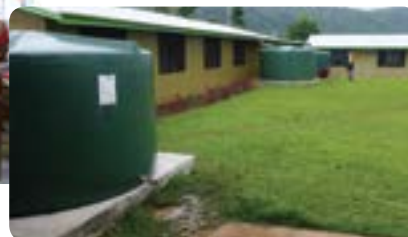
Patients at Namatanai hospital and (inset) the outside of the hospital showing installed water tanks.
